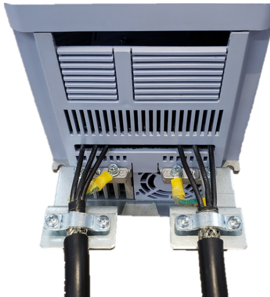
Figure 3.26: Detail of the motor cable shield connection
